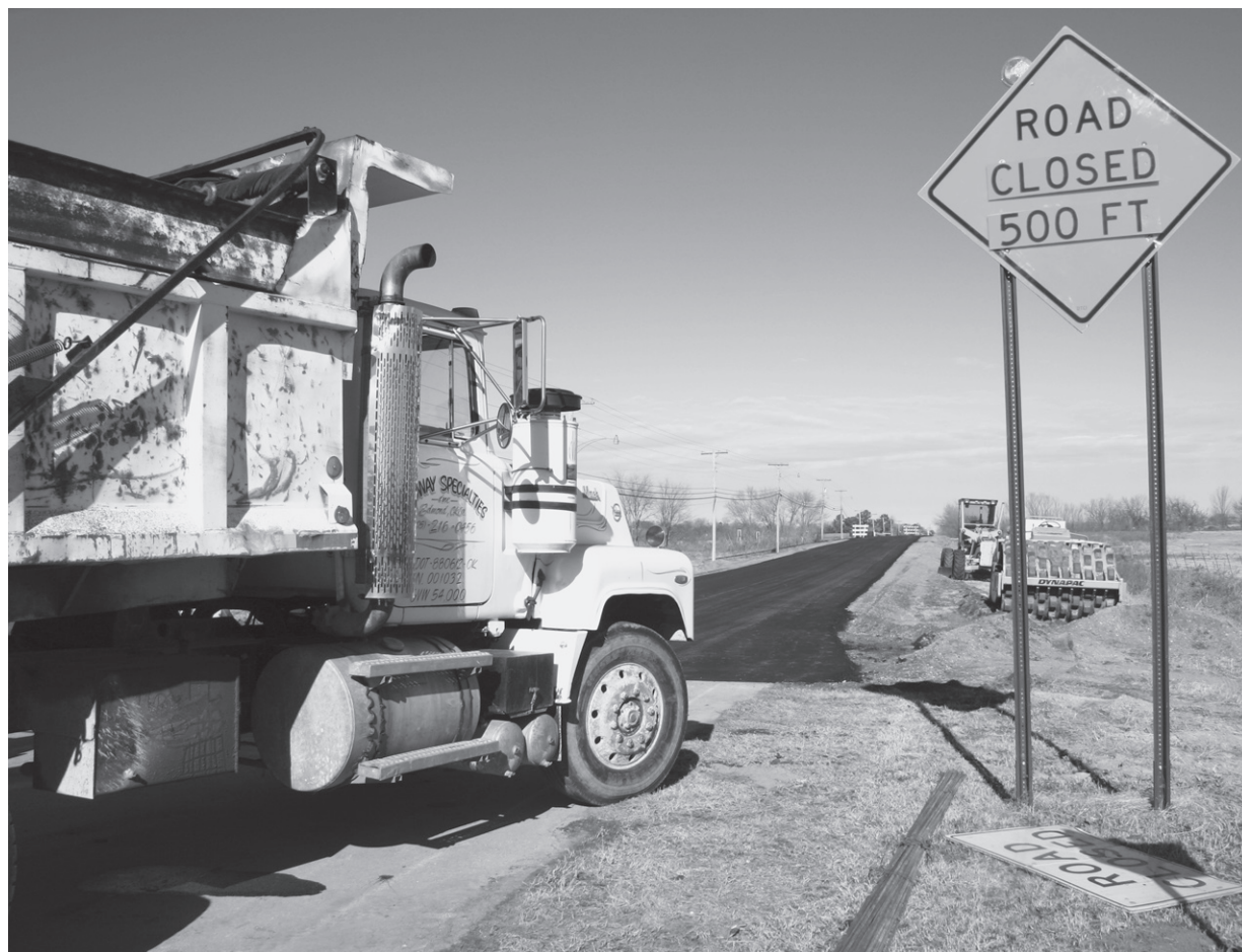
The bridge on Fourth Street is just one step away from completion. The bridge needs one more layer of blacktop before it will be open. The crew is waiting on the weather to warm up so they can place the layer of black top down and then the bridge will be open to traffic.
