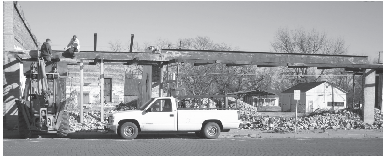
Demolition began recently on the old Miller Motors building located on the south end of Main Street. The building burned in January 1977 and is being demolished by Sebastian and David Geffre.
