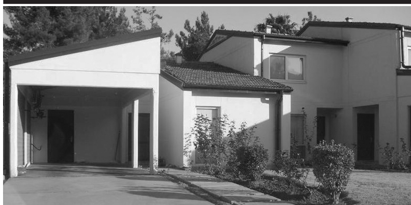
This is a part of a housing unit, only two of the three sections are shown here. The one to the far left is our house. It is a two bedroom, one bathroom house.
