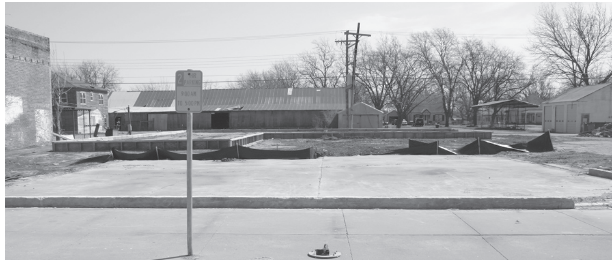
Dr. Robert Westcott and his staff will be relocating to Main Street. The new office is currently being built next door to the American Exchange Bank Mortgage office at 405 S. Main Street.
