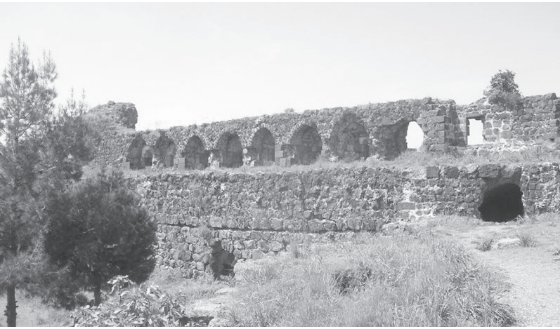
This is a shot of a section of the inner wall of Black Castle. This is the only section of the inner wall still standing.
