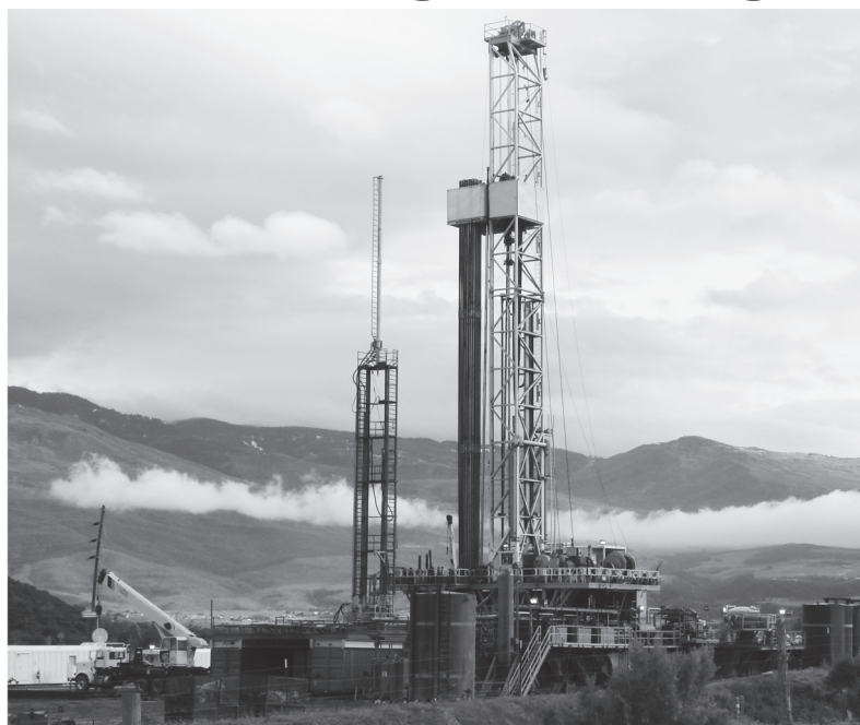
Troy's Versa-Rig is shown working directly behind a Helmerich and Payne FlexRig in Parachute, Colorado in the Piance Basin. His rig is directly behind the FlexRig.
