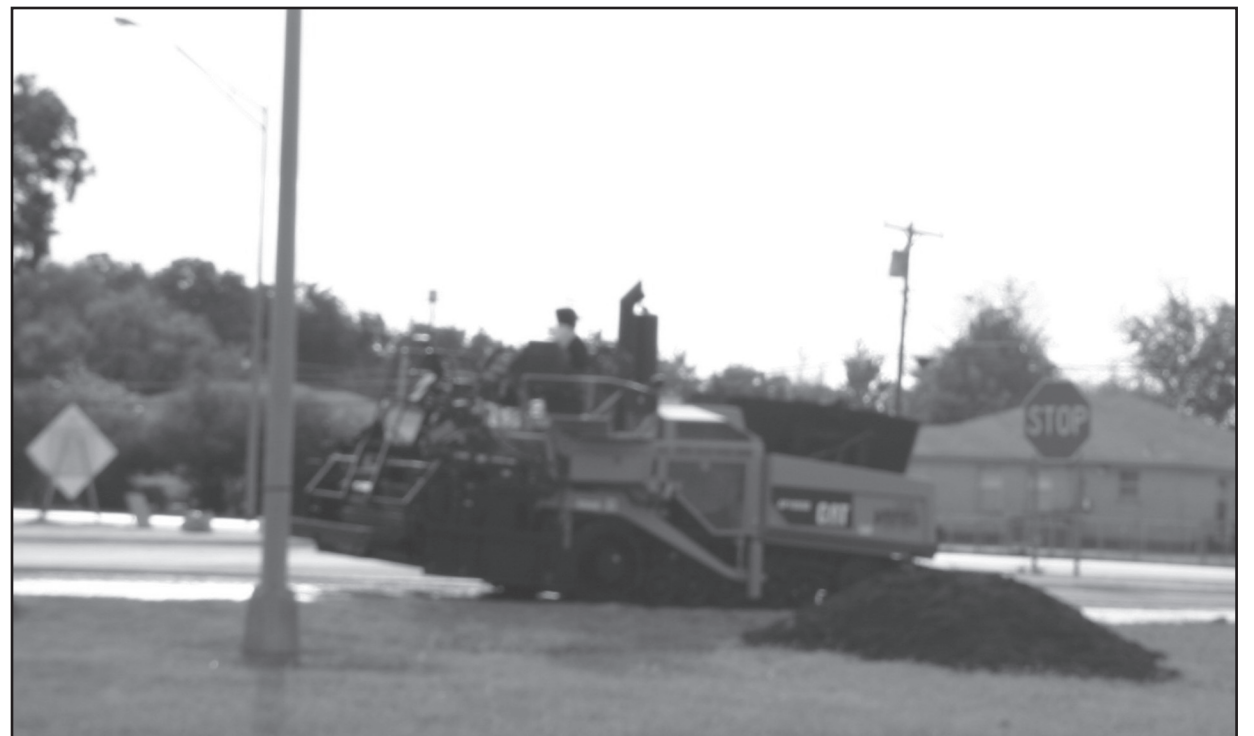
The Highways through Lindsay are being overlaid by the Oklahoma State Department of Transportation. The overlay is being done just east of Gas N Go through town to the bridge going north and just to the west entrance of Teran's Mexican Restaurant. The project is supposed to be done in eight days if the weather cooperates.
